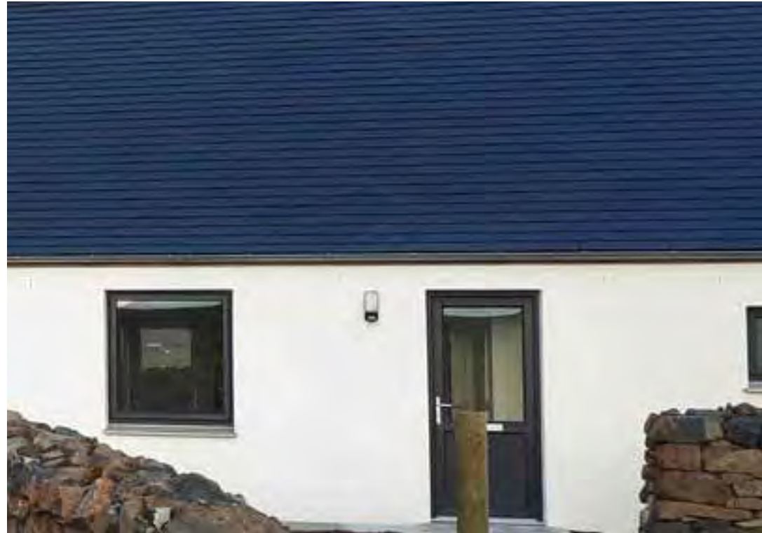
Slate roof and rendered walls are a typical combination of materials within Morayshire. The ambition to include dry stone walling is also in keeping with the area, and will be balanced against cost.
