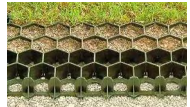
Permeable hard surfaces - helps to control water run off
