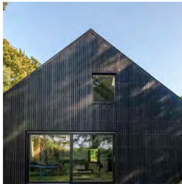
Timber cladding can be modified in a variety of ways, from paint through to heat and steam treatment to prolong the life of the product.
