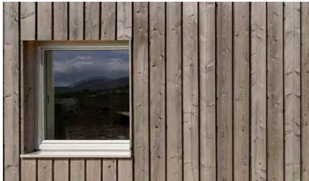
If left to weather, larch cladding, which is durable, will naturally grey over time. Careful detailing around windows and eaves prevents drips and staining.
