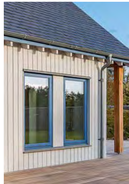
Timber cladding can be modified in a variety of ways, from paint through to heat and steam treatment to prolong the life of the product.
